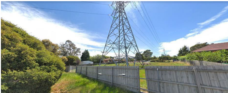
Figure 18 – Major electricity transmission lines traversing northern access point at Kiewa Street
