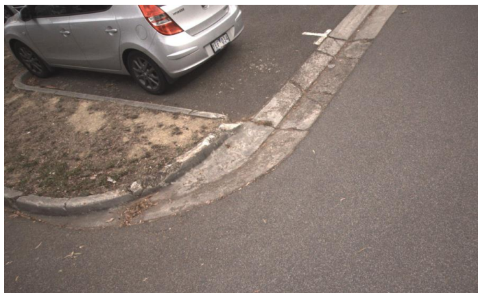
Figure 6 Snapshot of a very poor Kerb and channel in Anderson Park off-street carpark
