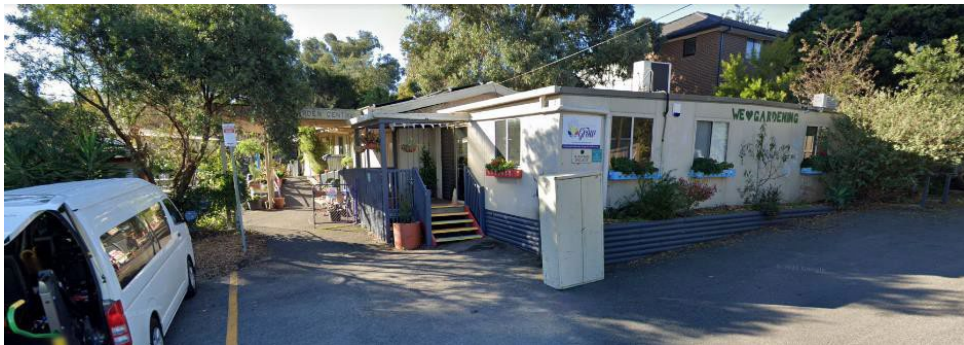
Figure 9 – KHG Office Building (shown in Figure 3 as Building 7)
