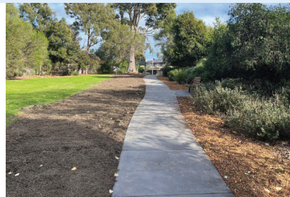
Tolsoy Footpath Construction
