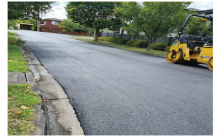
Saxonwood Drive Resealing Works
