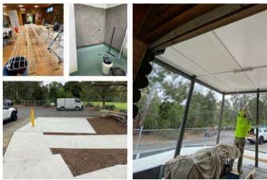
Finns Reserve Scout Hall refurbishment in progress
