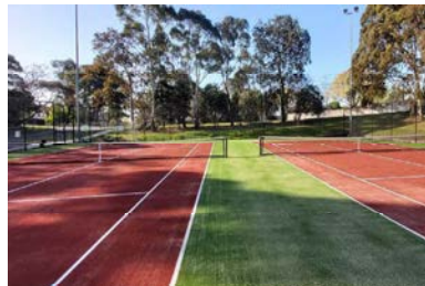
Park Orchards Tennis Club Courts synthetic resurfacing, new fencing, and net posts/nets.
