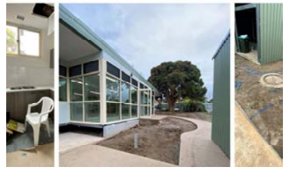
Tunstall Square Kindergarten building nearing completion
