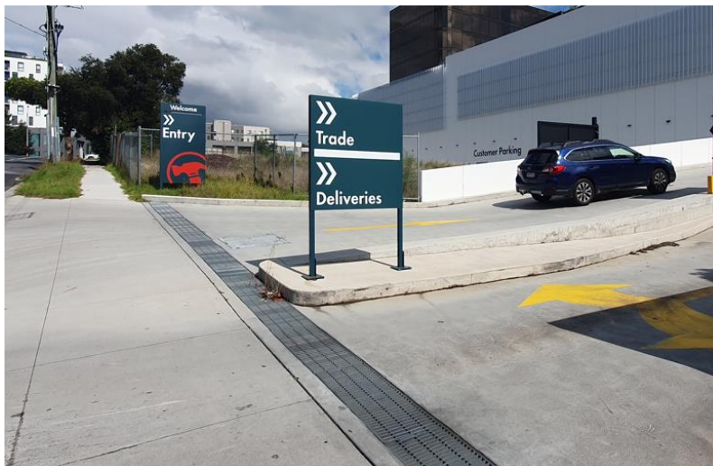
Image: Rear ramp access showing signage affects drivers sightlines
