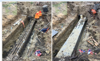
Everard Drive, Warrandyte (in progress)
