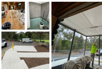
Finns Reserve Scout Hall refurbishment in progress
