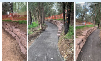
Jumping Creek Road Reached detailed design stage, with recreational trail works in progress
