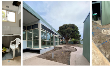
Tunstall Square Kindergarten building nearing completion with landscaping to follow
