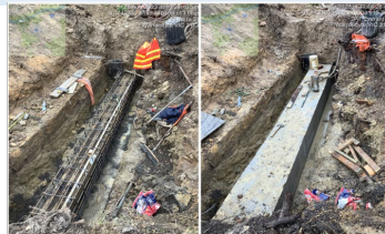
Everard Drive, Warrandyte (in progress)
