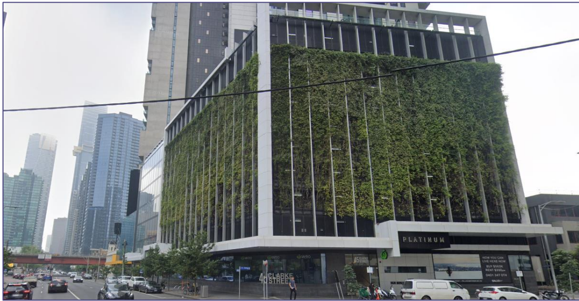
Figure 1 – Green wall example (Source: Google Streetview, image dated Dec 2022).
