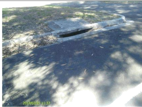
Damaged Pit Lintel
