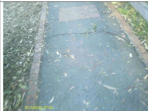
Pavement Cracking
