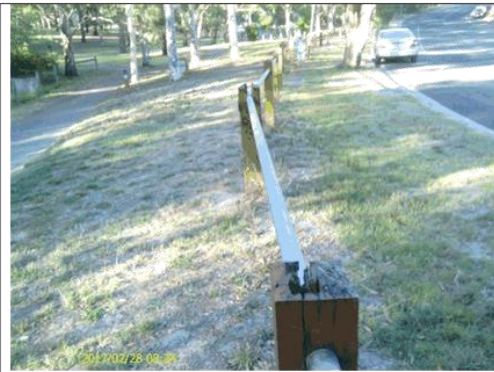
Damaged Bollards
