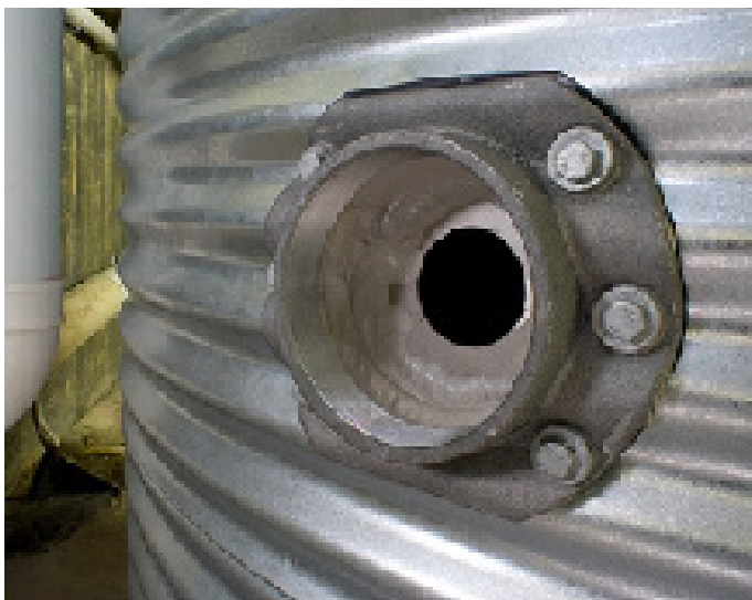
Figure 5 - Rainwater tank orifice installations
