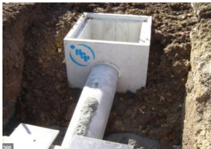
Figure 3 - Outfall drain construction
