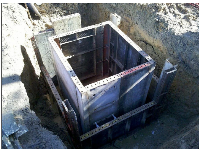
Figure 2 - Junction pit construction
