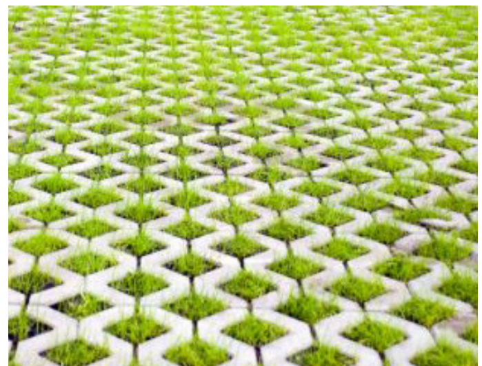
Figure 14 - Grass and gravel pavers
